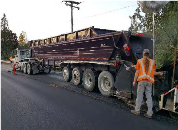
Figure 4. Flow Boy truck delivery to Shuttle Buggy MTV.
