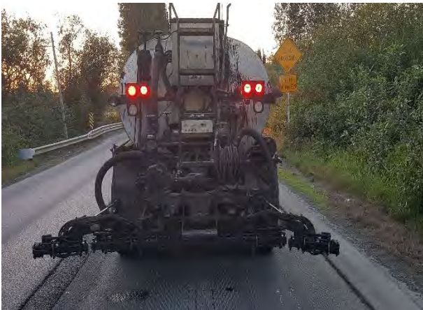
Figure 2. Bearcat distributor on milled surface.
