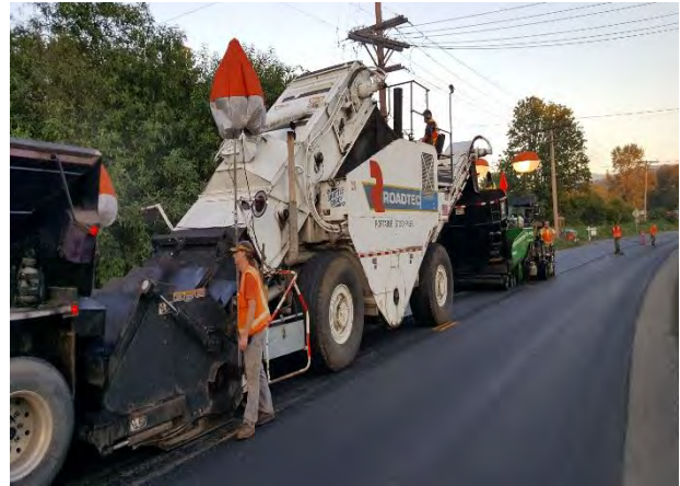
Figure 5. Shuttle Buggy MTV delivering HMA into hopper on the paving machine.
