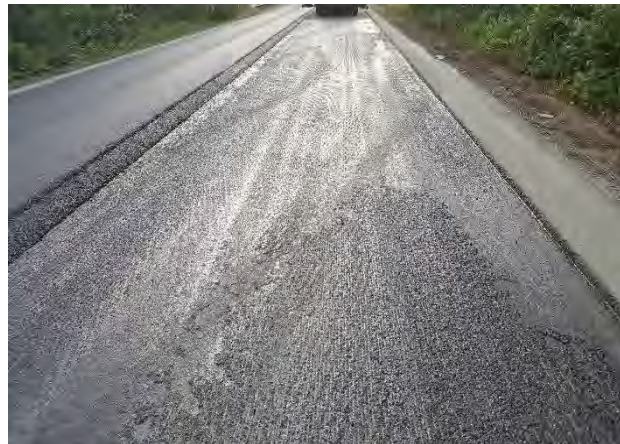
Figure 3. Milled surface with CSS-1 tack coat.
