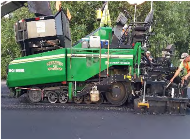
Figure 6. Barber Greene paver with storage hopper.
