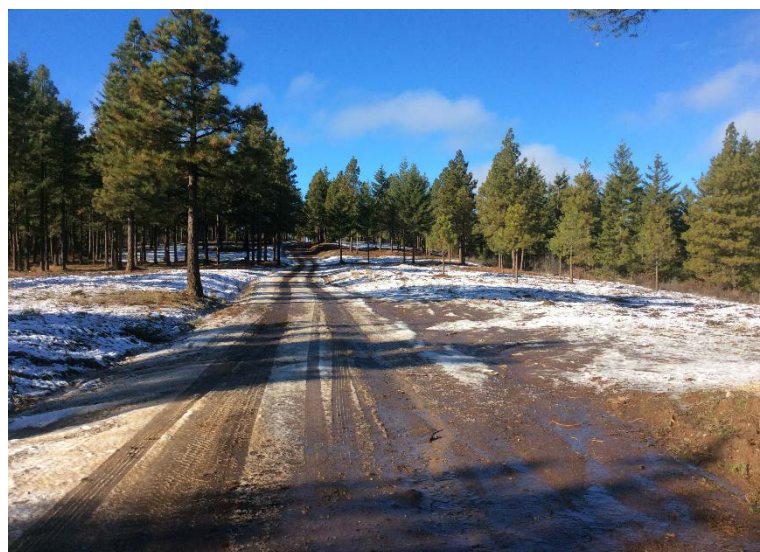
A shaded fuel break along a forest road in eastern Washington; DNR has planned over 9 miles of shaded fuel breaks in the next biennium
