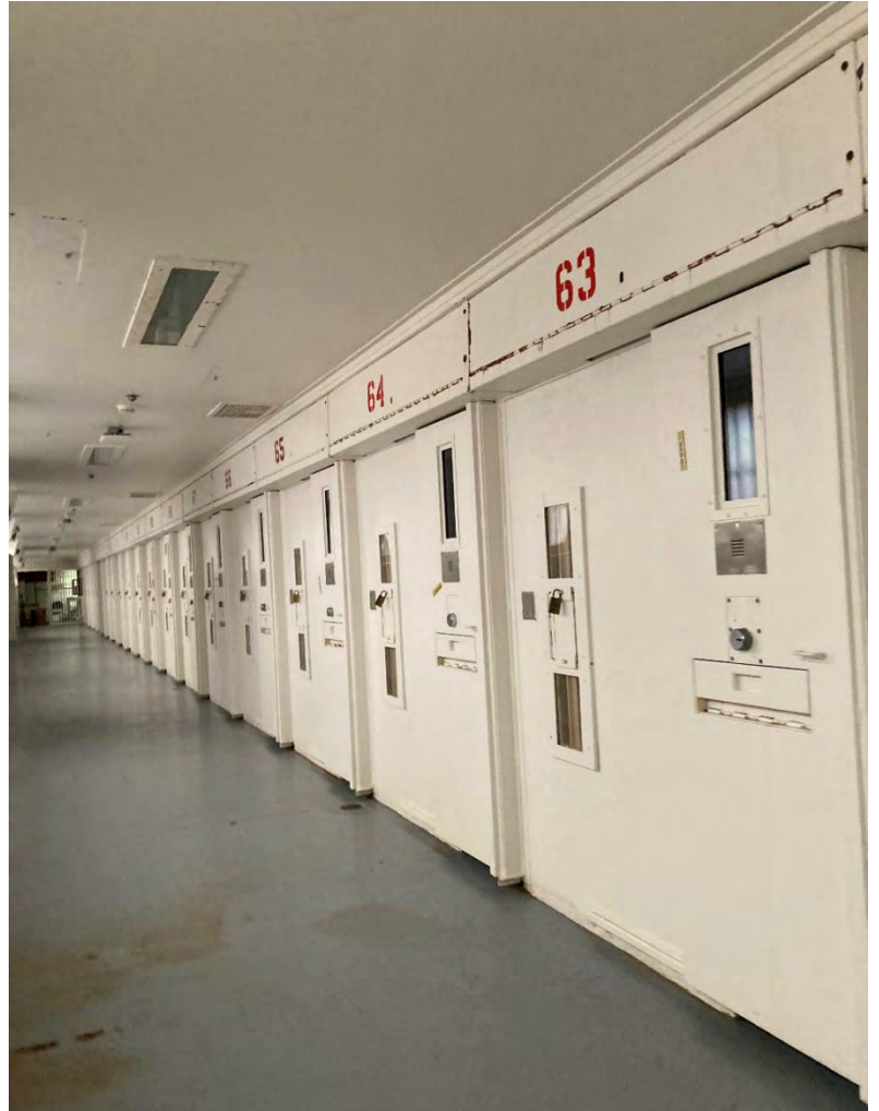
Former solitary confinement cells at Washington State Reformatory at Monroe Correctional Complex
