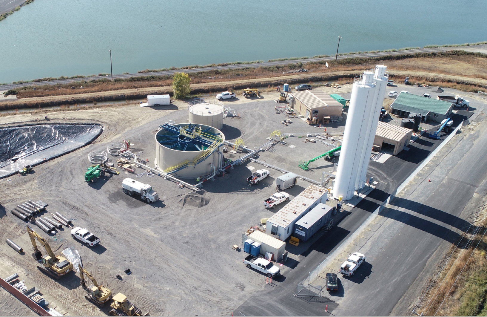
Construction of the city of Quincy's Industrial Wastewater Reuse Facility
