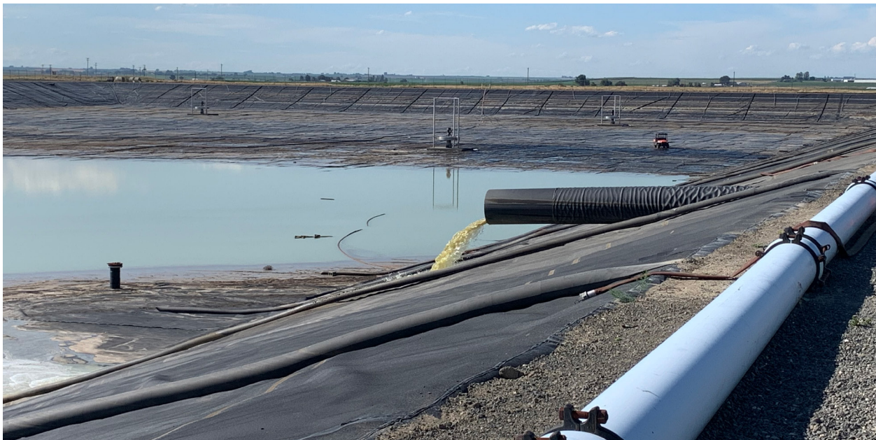
Waste flow into retention pond that will be used to harvest algae
