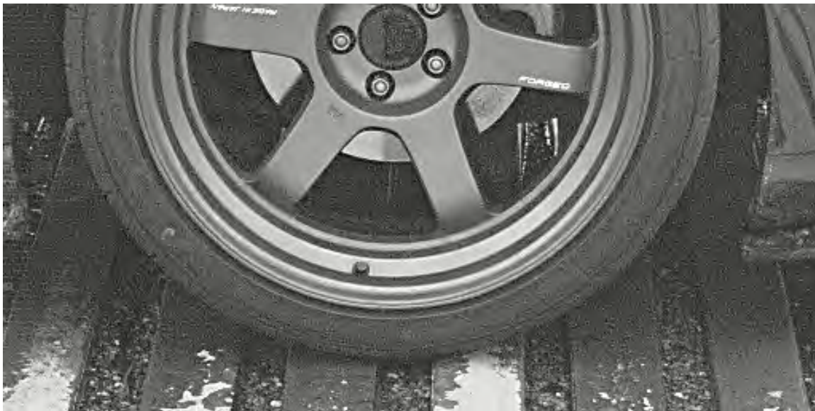
Figure 5-17 Frame from high-speed video recording of a Scion sports car front tire passing over east-side large expansion joint center beams.
