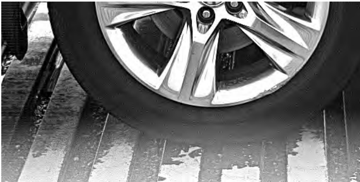
Figure 5-19 Frame from high-speed video recording of a Toyota Tundra front tire passing over east-side large expansion joint center beams.
