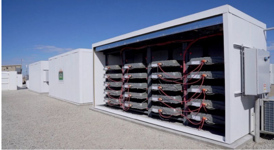
Figure 4. B2U’s UL certified EV Pack Storage (EPS) System enables the use of EV battery packs without reconfiguration in large scale energy storage.
