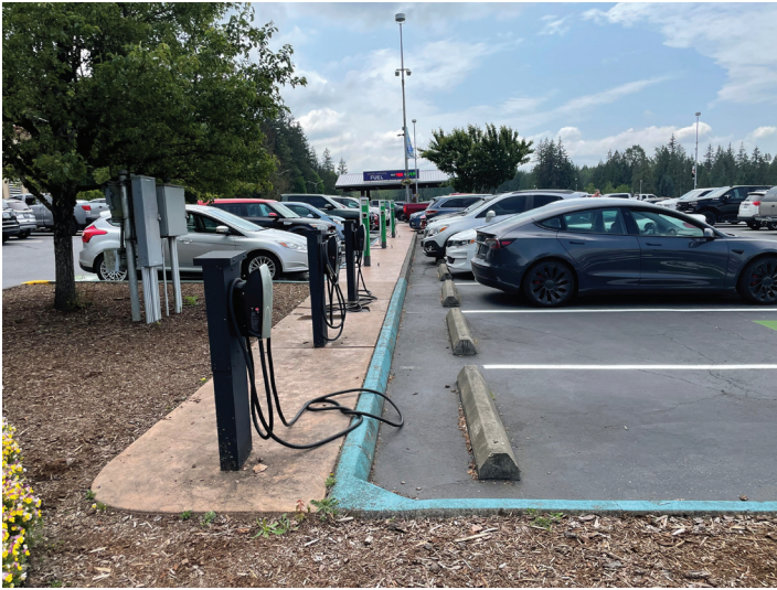
With GTP assistance, the Stillaguamish Tribe of Indians developed a $2 million plan to install Level 2 and DCFC stations at the Angel of the Winds Casino near Arlington.
