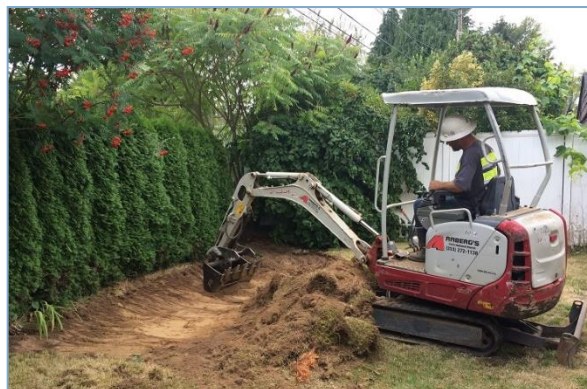
Photo 3: Contractors removing the contaminated soil at a home in Tacoma.
