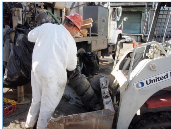
Photo 12: Worker installing a remedial well at the former Lilyblad property.
