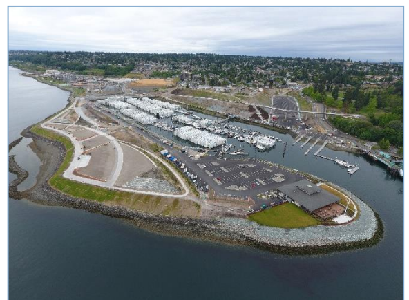
Photo 5: Point Defiance Trails project during construction. Photo courtesy of Atkinson Construction.
