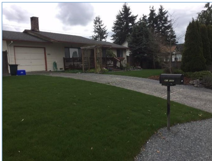
Photo 2: Property after cleanup and contractor maintenance is complete.
