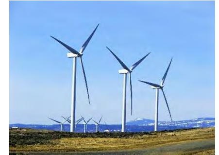
IMAGE SHOWS WIND TURBINES ON STATE-TRUST LANDS. SOURCE: WA STATE DNR
