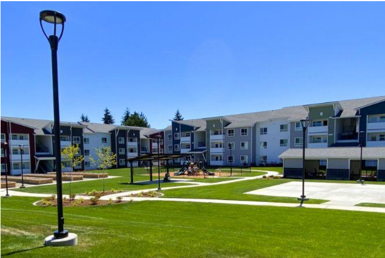
Novo on 52nd, in Lynnwood, replaced the Whispering Pines affordable housing complex with 242 new affordable units. Photos provided by the Housing Authority of Snohomish County.
