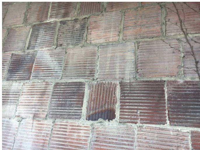
Left: Stone Masonry. Right: Detail of Hollow Clay Tile wall. Blocks are approximately 8"x8".
