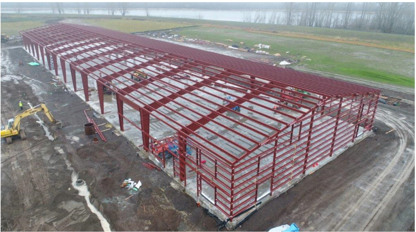
Port of Camas-Washougal Building 18
