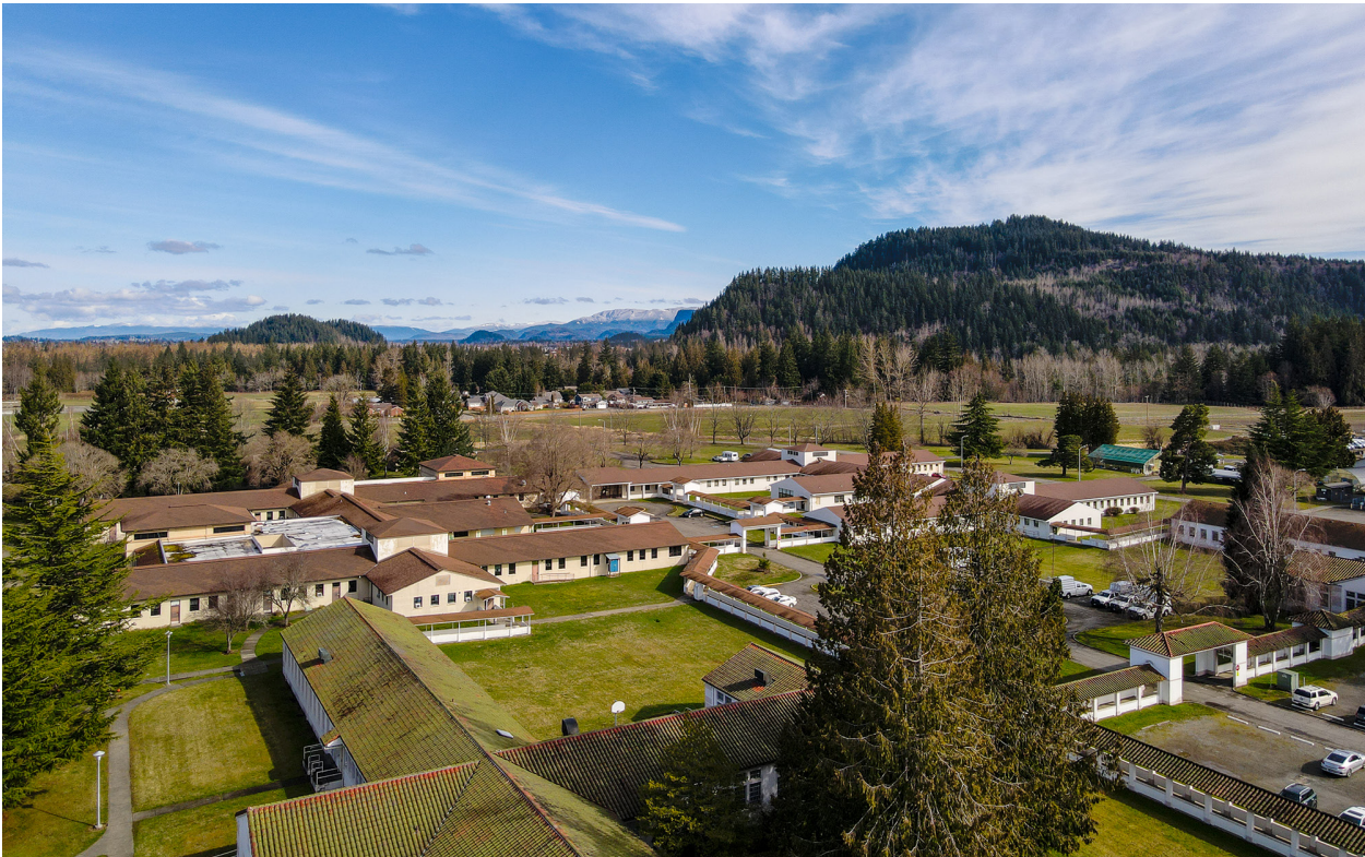
Figure 1 Aerial view of northern portion of Rainier School 2023
