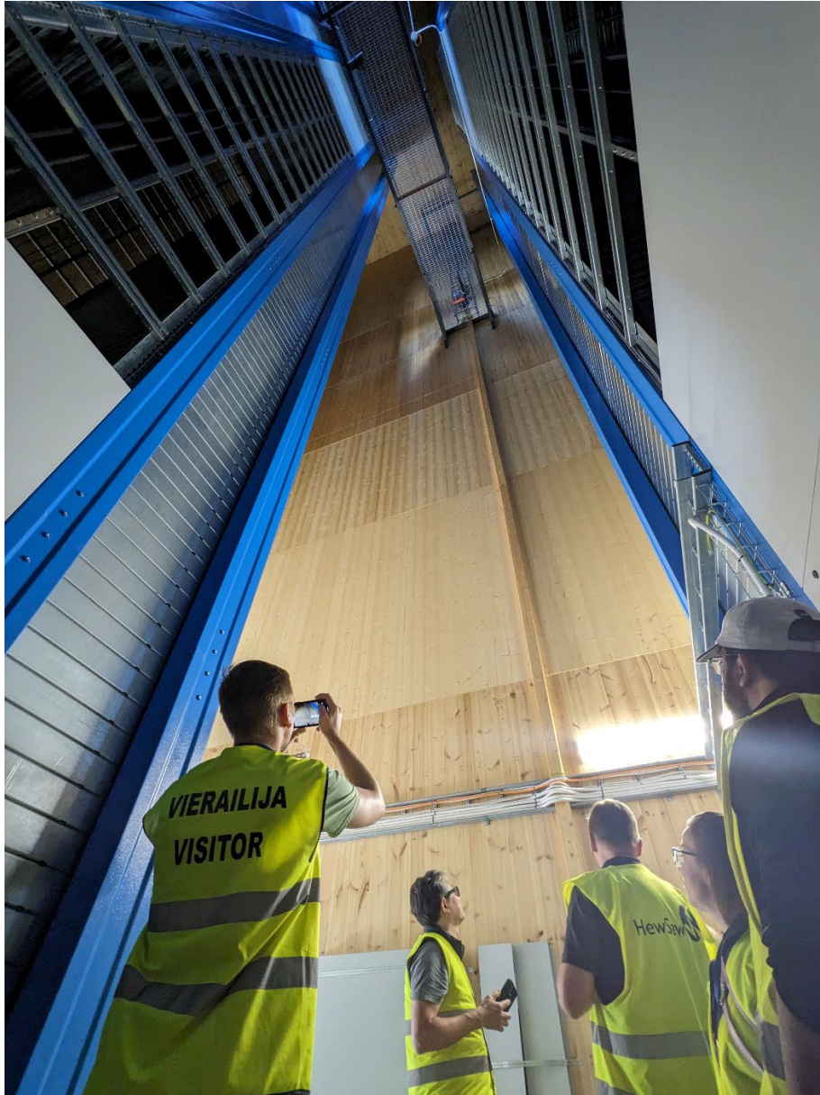
Examining a multi-story storage tower at HewSaw (Finland) made from CLT panels from Vaagen Timbers (Washington)
