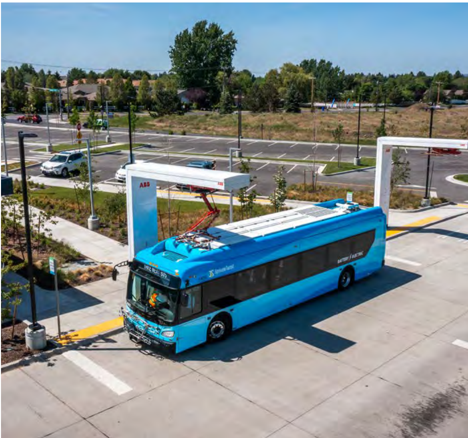
Charging up one of Spokane Transit's battery-electric buses.
