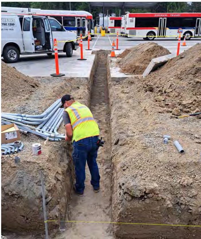
Installing new infrastructure for battery-electric buses.
