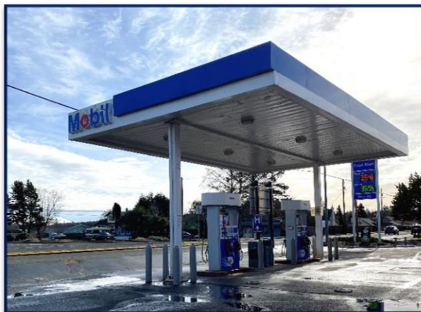
The canopy and fueling dispensers prior to cleanup and construction.
