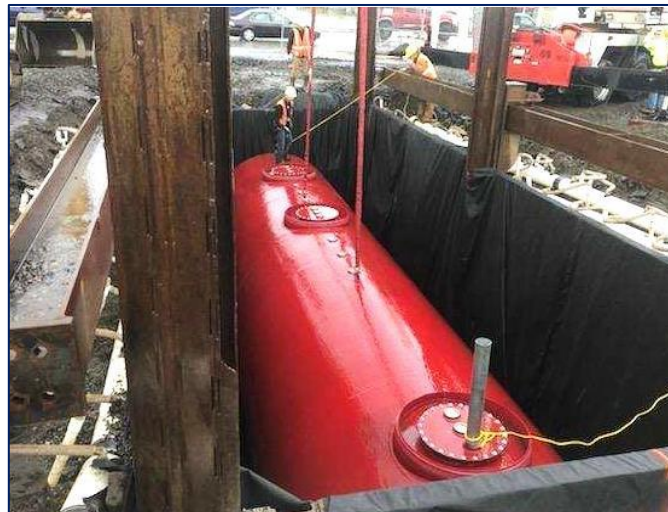
Installation of new multi-chambered UST. Photo credit: Vertex.
