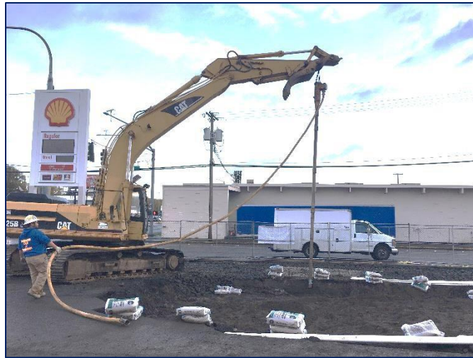
Installation of wells for groundwater extraction. Photo credit: Vertex.
