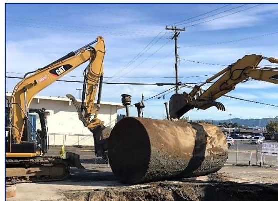
Removed diesel tank. Photo credit: Vertex.
