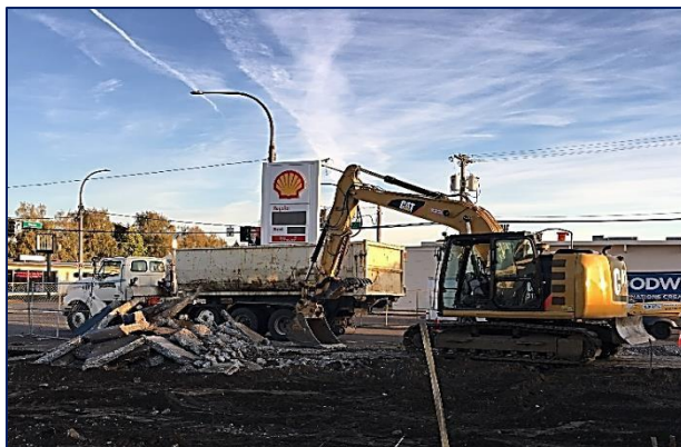
Removing concrete above USTs. Photo credit: Vertex.
