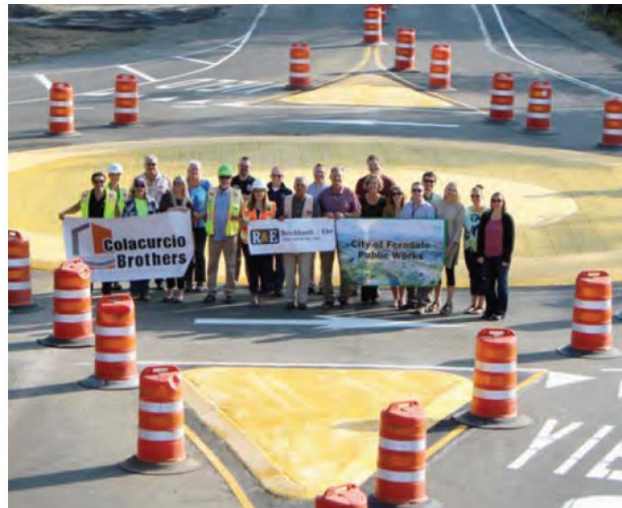
Roundabouts continue to reduce the potential for fatal and injury crashes throughout Washington. From 2004 to 2017 no bicyclist or pedestrian fatalities were reported at roundabouts in Washington state.
