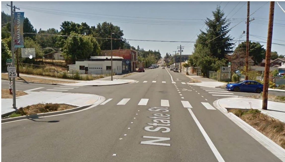
An effectively designed intersection in Bellingham, WA that has curb extensions, ADA ramps, crosswalks and a connection to a nearby trail system.
