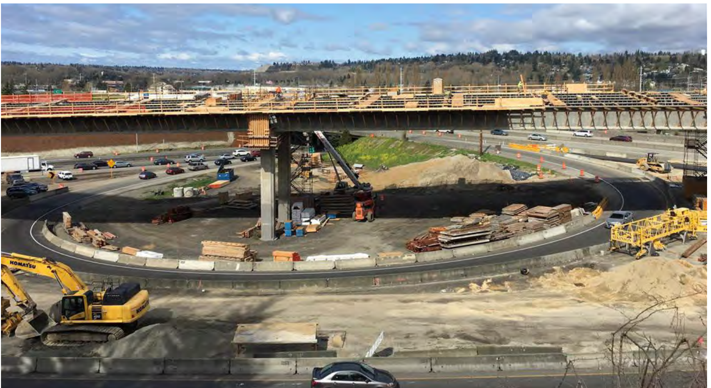
I-405/SR 167 Interchange Direct Connector design-build project under construction in summer 2018
