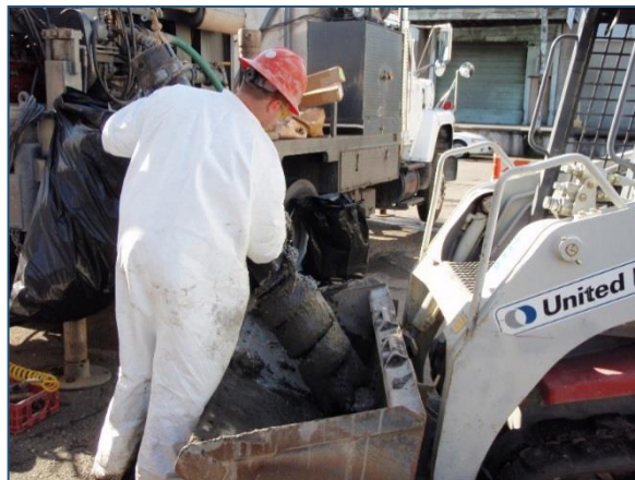
Photo 12: Worker installing a new remedial well at the former Lilyblad property.
