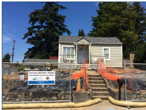
Photo 3: Contractors removed the top 18 inches of contaminated soil at a home in Tacoma.
