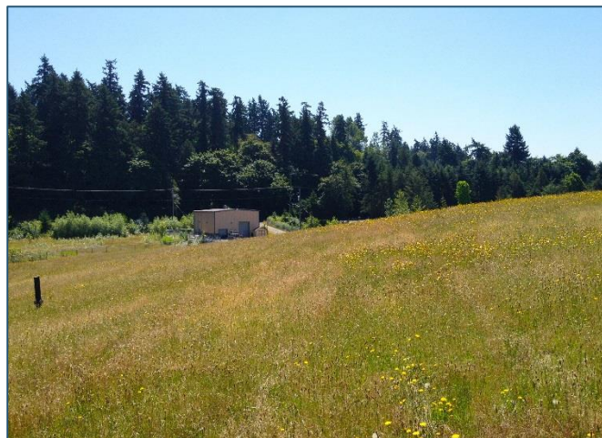
Photo 8: The 11-acre landfill with cap and vegetation at the B&L Woodwaste site.
