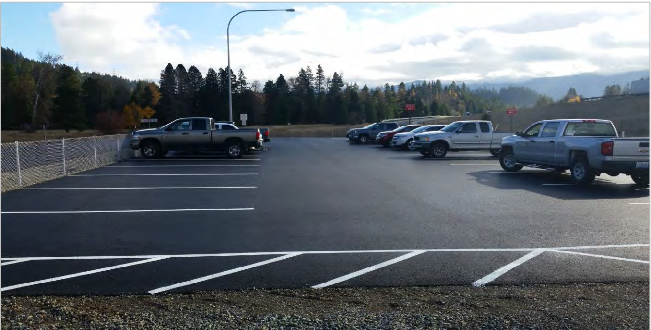
Kittitas Park and Ride (I90 – exit 78) Completed October 2016
