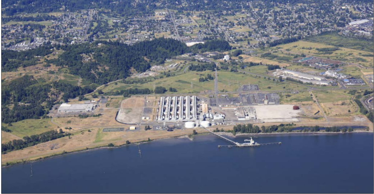
Figure 9: The former Reynolds Aluminum Smelter Site includes more than a mile of Columbia River frontage in the Longview industrial area. The cleanup plan finalized in 2018 will support economic redevelopment and protect adjacent aquatic resources. Photo credit: Washington State Department of Ecology.
