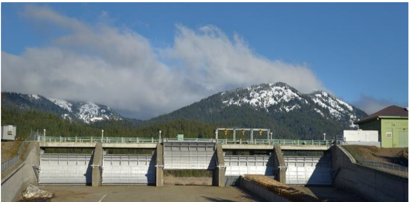
Completed Cle Elum Pool Raise 3' Radial Gate Expansion
