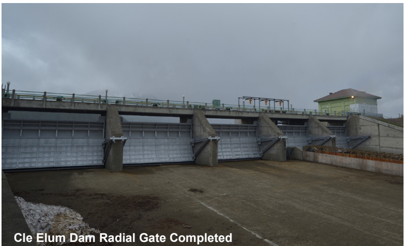
Cle Elum Dam Radial Gate Construction
