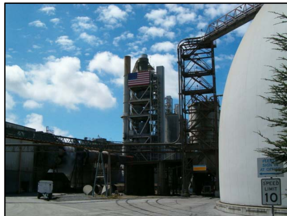
Ash Grove cement kiln in Seattle
