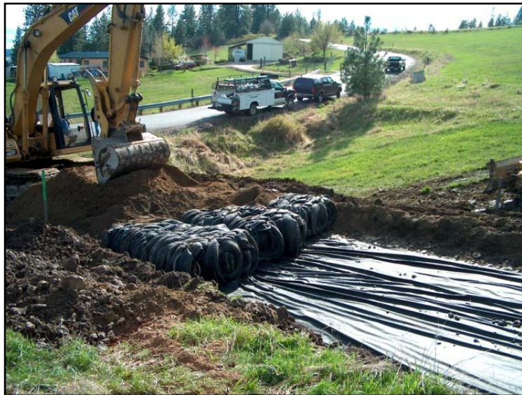
Tire bales used for road base in Spokane County
