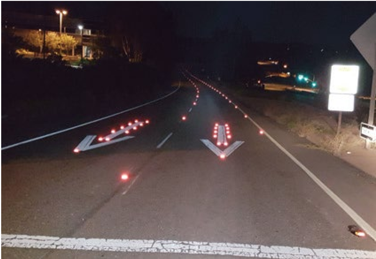
Figure 12: Two-way Retroreflective Raised Pavement Markers
