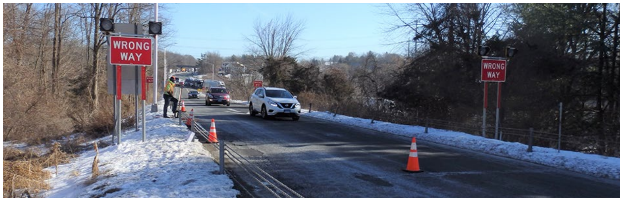
Figure 10: CTDOT Flashing-beacon Wrong-way Alert Signs
