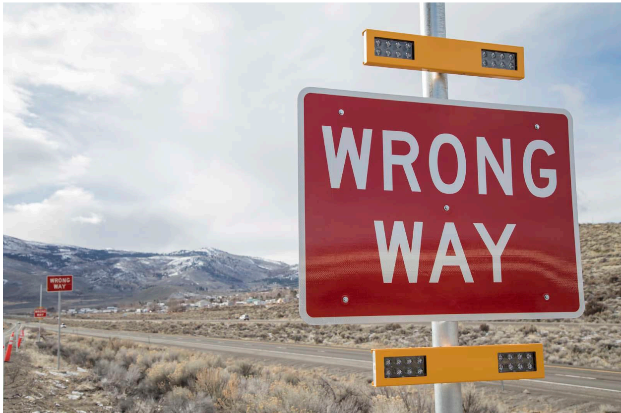
Figure 11: NDOT Wrong-way Driver Alert Signs
