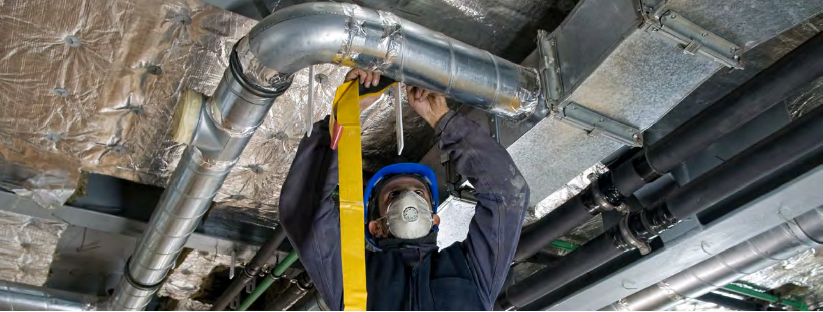
Worker wrapping an HVAC air duct with foil tape. 1905HKN/iStock
