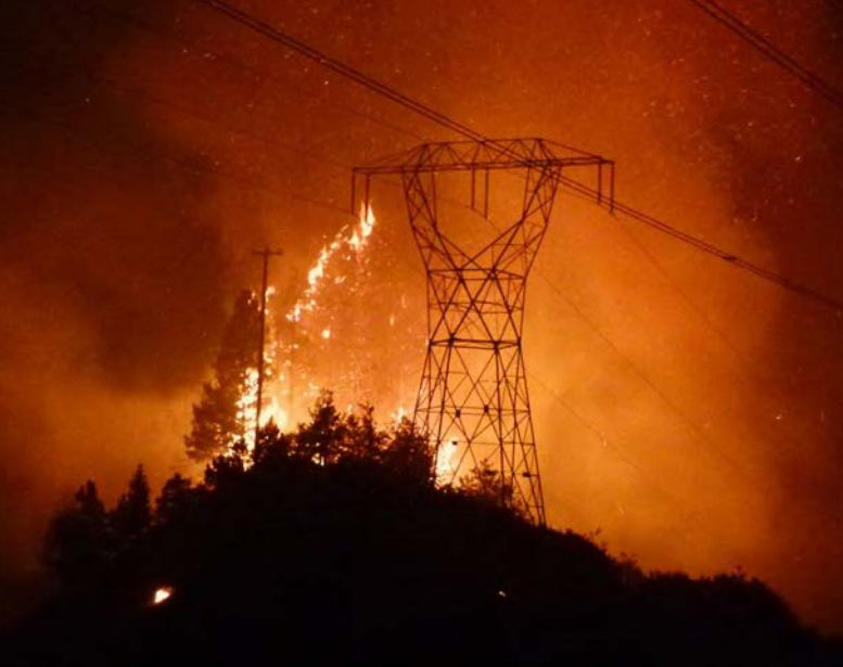
Fire threatening power lines running along US 97 in Washington State. WA State Department of Transportation
