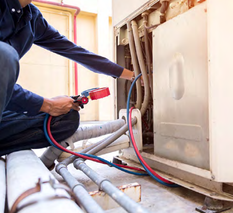
Technician measuring air conditioning equipment.
