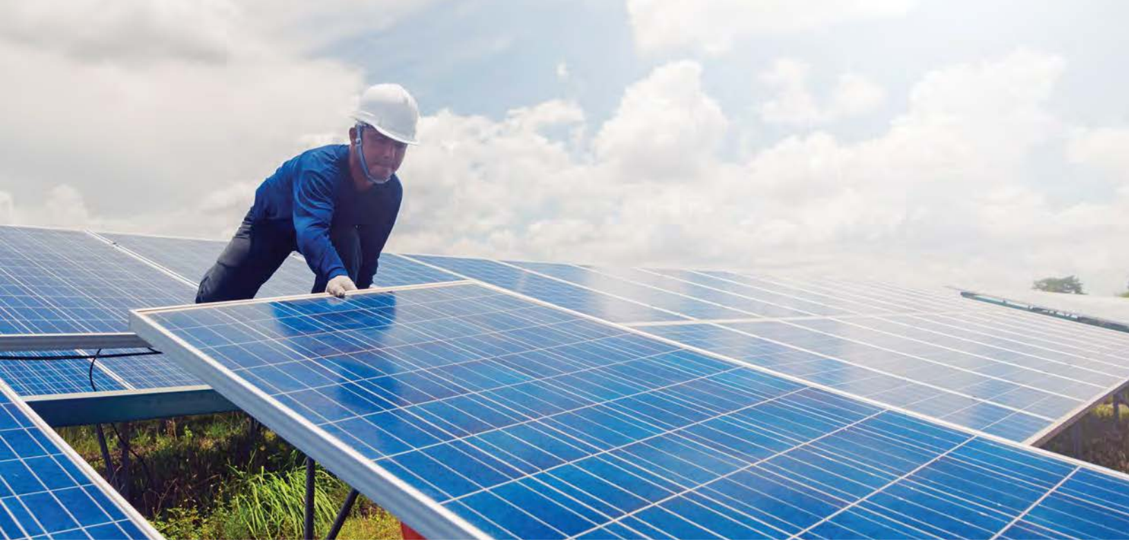
Engineer installing solar panel.
