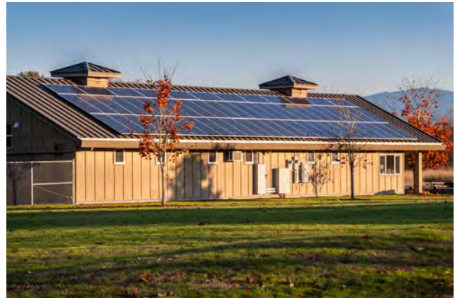
Solar panels on roof of North Utility Building at Marymoor Park, WA.
