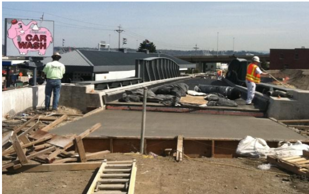
Sound Transit, Lakewood to Tacoma Commuter Rail D to M Street waterproofing Pacific Ave and retaining wall construction
