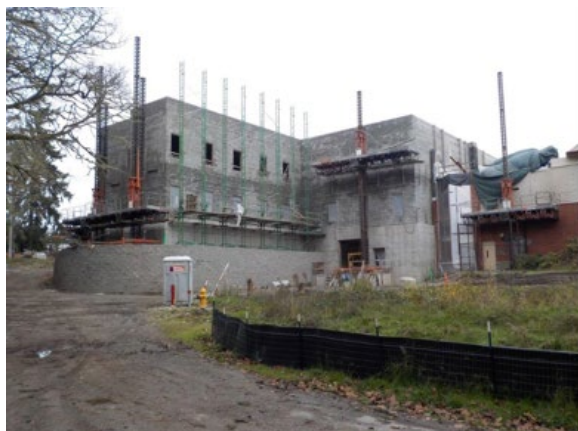
Exterior CMU walls
