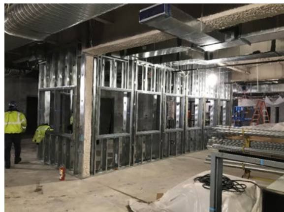
Interior framing at Nurses Station
