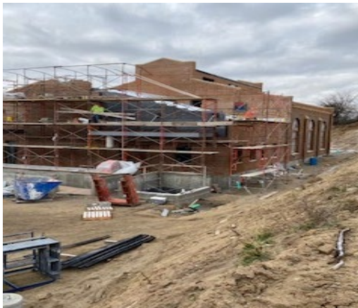
Exterior brick veneer
