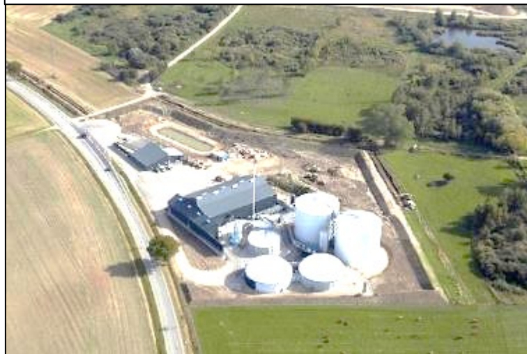
Photo 1: Solrod Biogas A/S Plant
