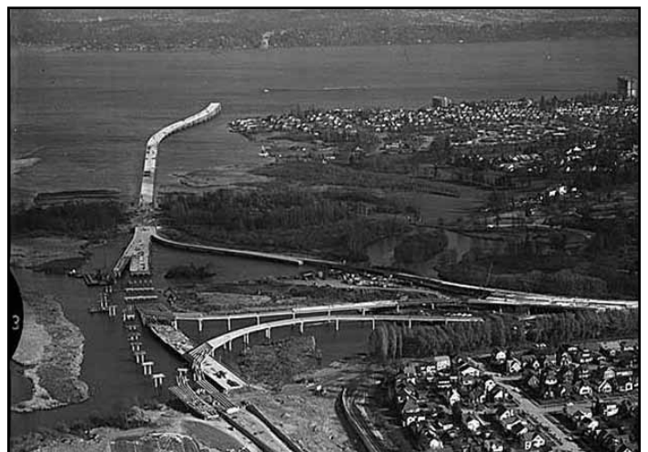
Construction of the existing SR 520 bridge west approach section in 1962.
