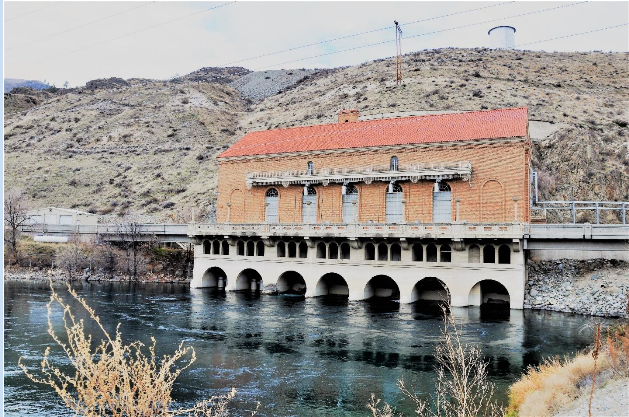
Chelan River Hydroelectric Facility on Chelan River
