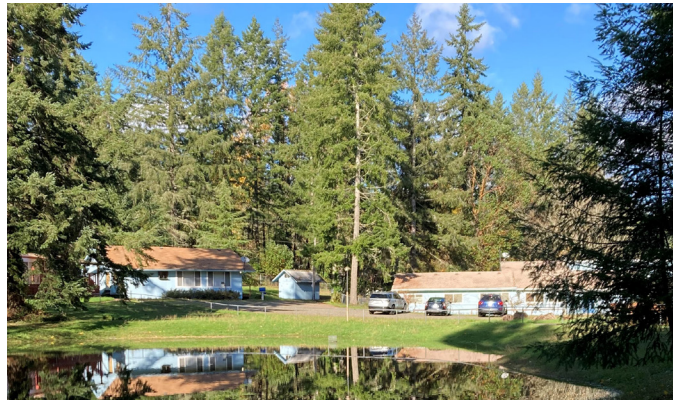
Stabilization, Assessment and Intervention Facility located in Pierce County
