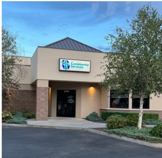
BHF-funded facility in Pasco
