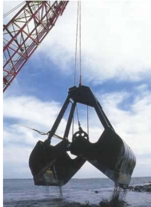
Open Water Dredging with Clamshell Crane
