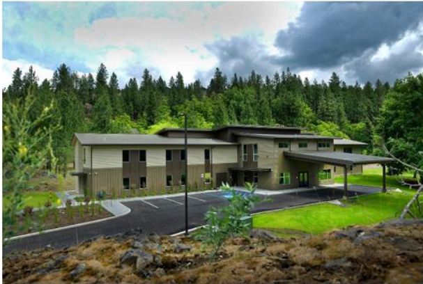
Commerce BHF-funded facility in Spokane Valley, WA
