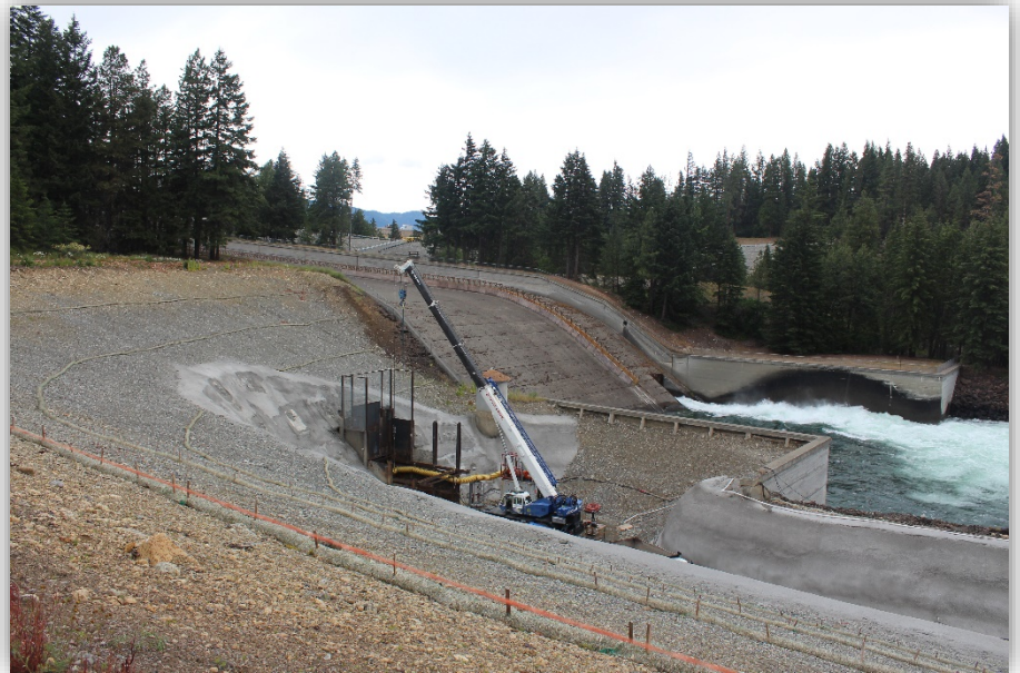
Cle Elum Fish Passage Construction, August 2019
