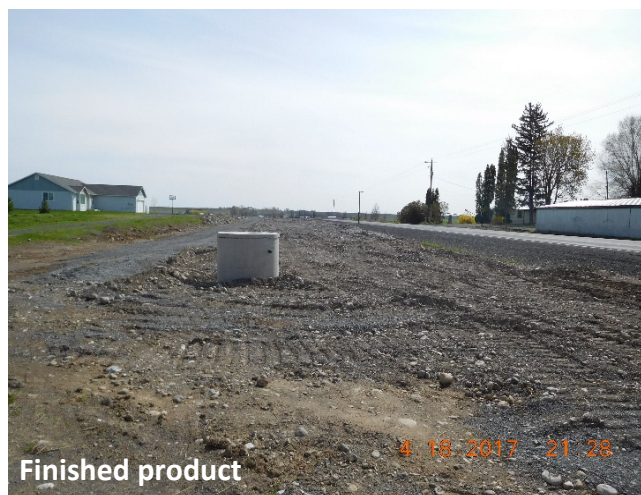
Quincy Columbia Basin Irrigation District Water Conservation Piping Project Photos
