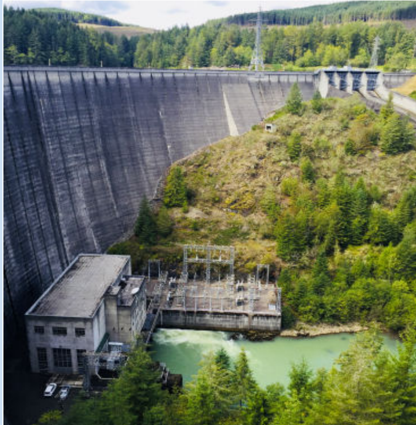
Alder Dam on the Nisqually River
